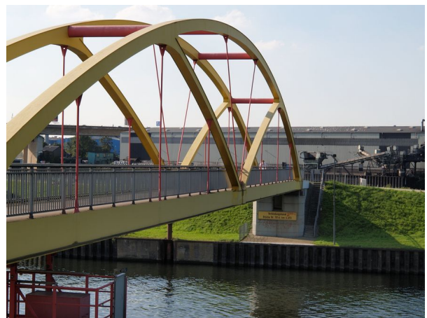
Bridge over Ruhr canal at Duisburg
