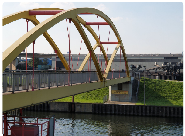
Bridge over Ruhr canal at Duisburg
