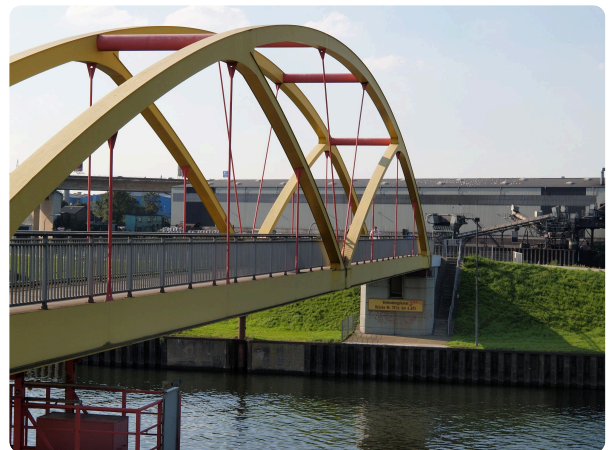
Bridge over Ruhr canal at Duisburg
